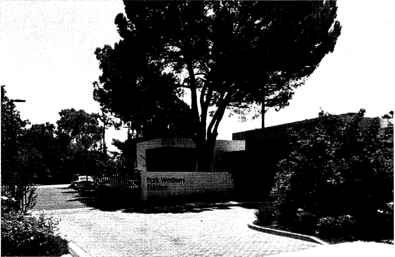
Park Western Estates (SDG LIHTC Renovation) San Pedro, CA
