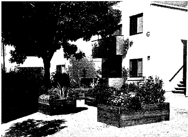
Woodman Nordhoff Apartments (SDG LIHTC Renovation) Los Angeles, CA
