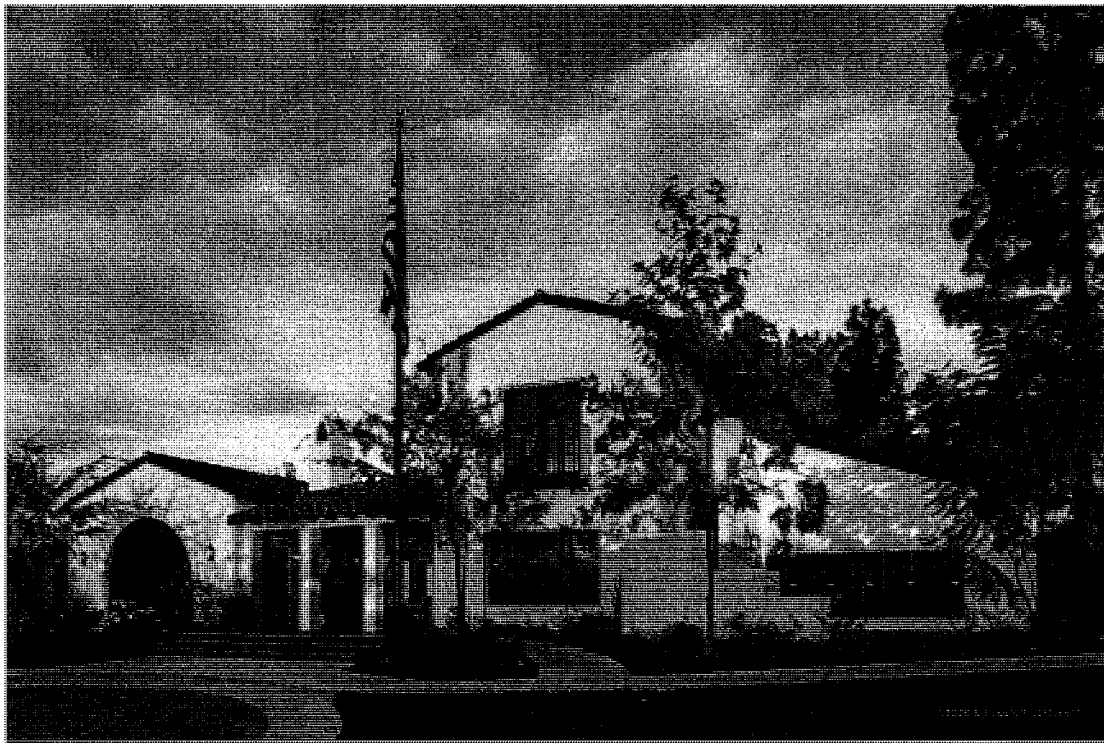
La Villa Puente Apartments – Los Angeles, CA, New Construction Example of Clubhouse
